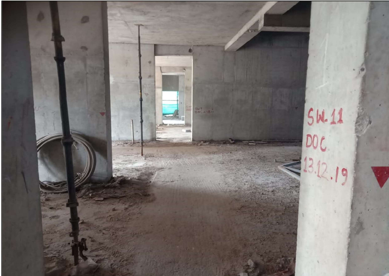
Ground Floor works under progress
